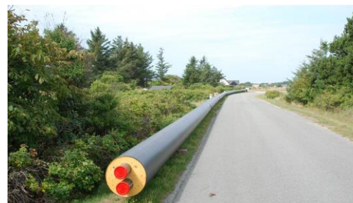
Fjernvarmerør – Twin-pipe. (Logstor, 2018)
